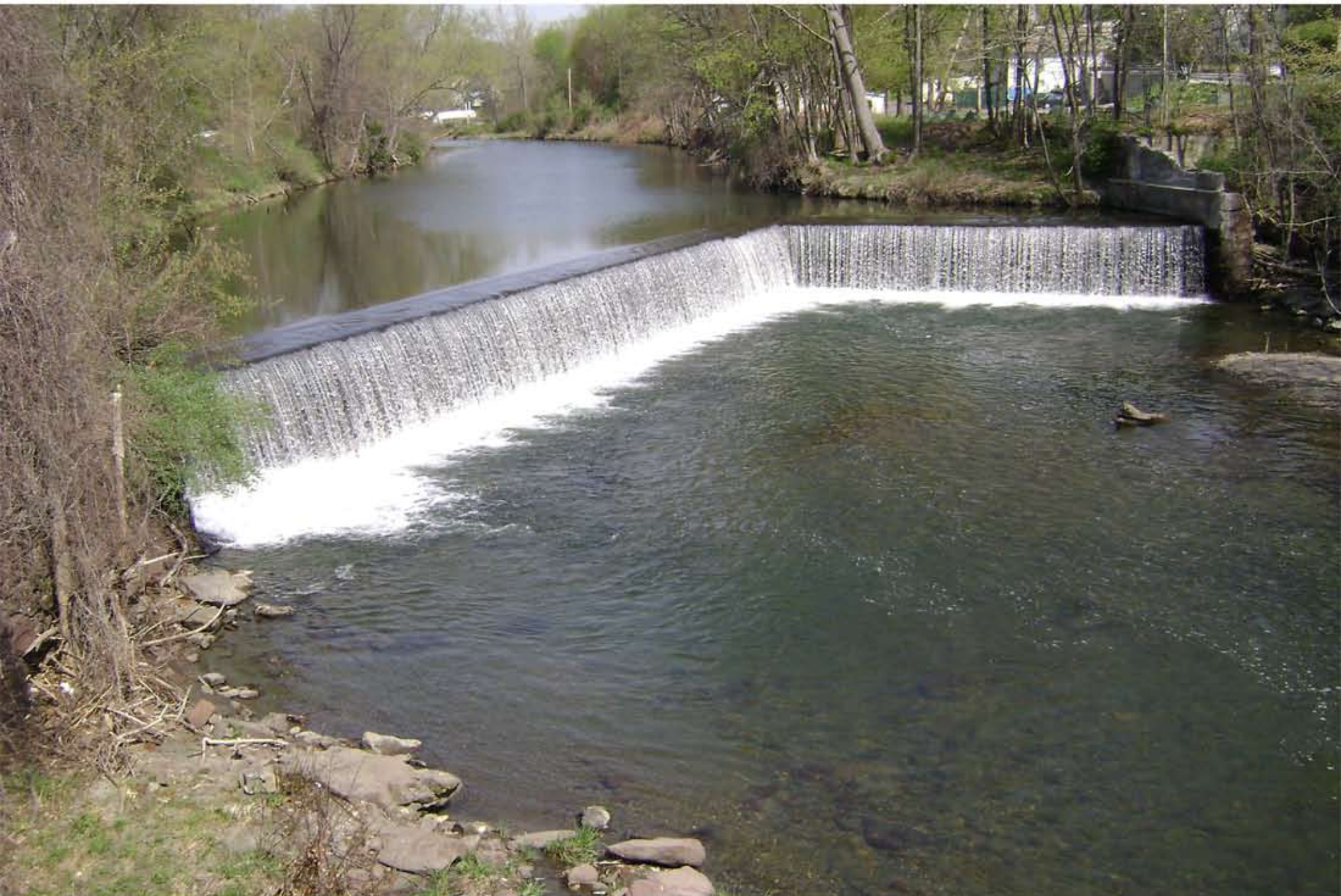
WILEY AND RUSSELL - ACTUAL VIEW OF EXISTING DAM
