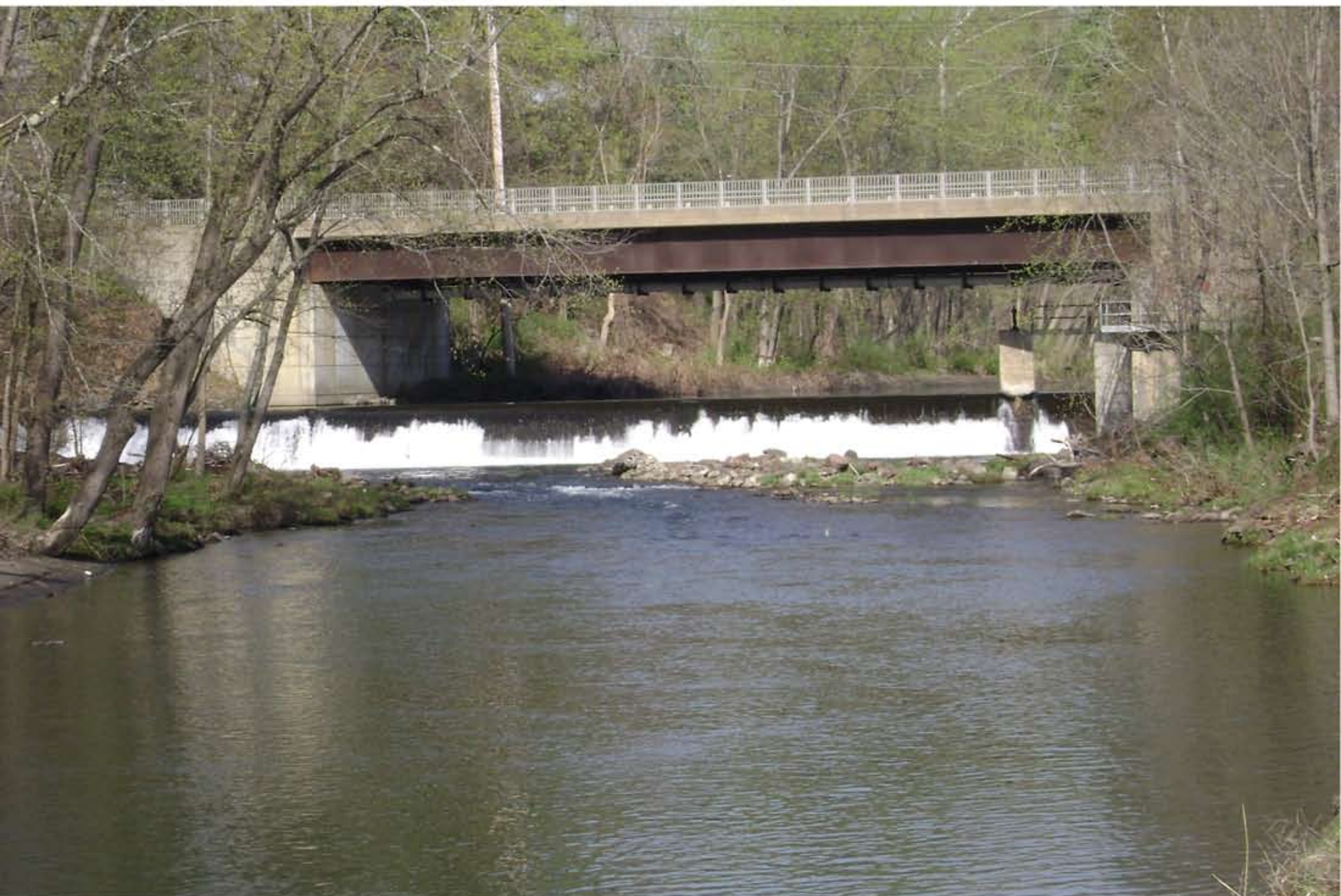
MILL STREET- ACTUAL VIEW OF EXISTING DAM
